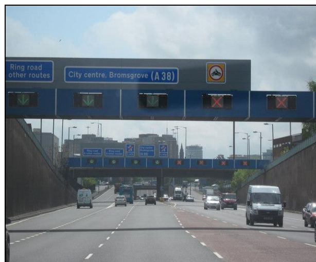
Slika 26. Autocesta A38, Birmingham, Engleska (Aston expressway)
