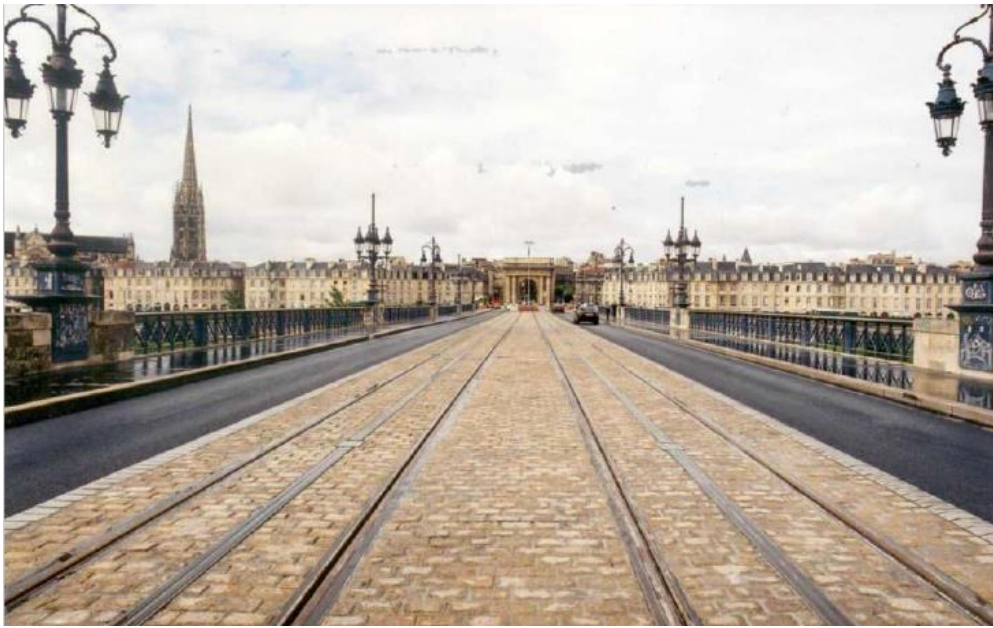
Figure 4 Estetic of Pont de pierre bridge after implementation of APS
