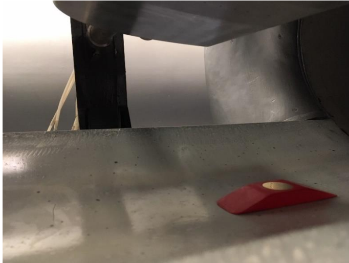
Figure 6- Existing element at the tunnel.
