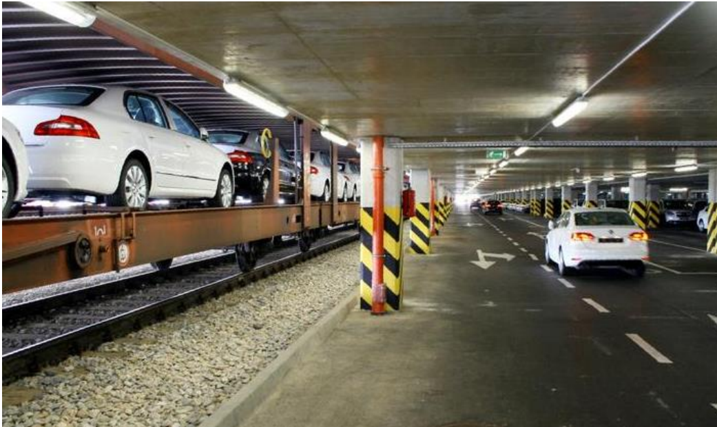
Slika 19. Car and RO-RO terminal u luci Koper
